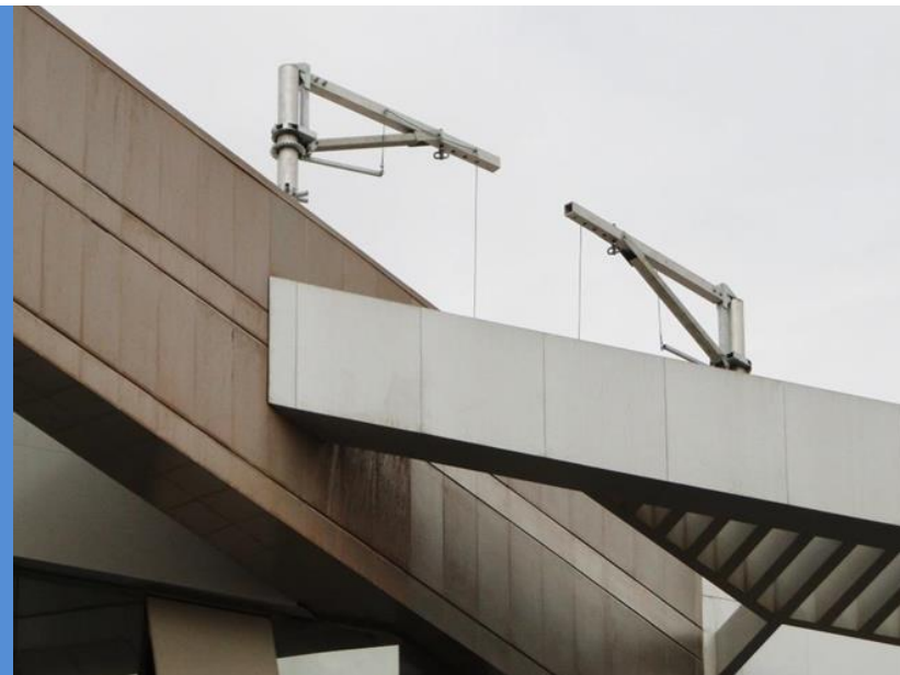
3 and 5 m mesh cladded Light Weight Stage for permanent installation with Alpha 500 hoists, Sky Locks, wire winders and rotatable davit arms.
