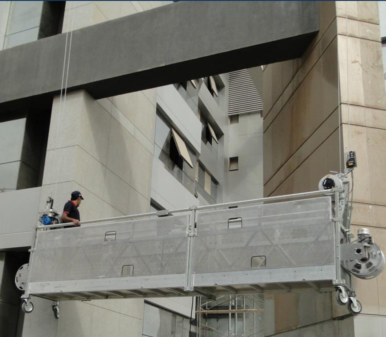
5 meters mesh clad Light Weight Stage with Alpha 500 hoists, Sky Locks and wire winders
